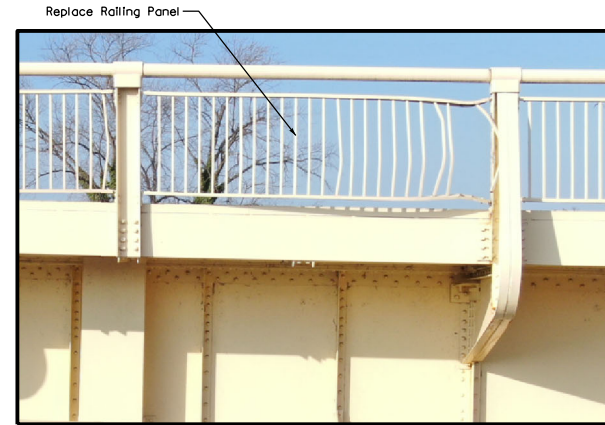
BRIDGE HANDRAIL REPAIRS (Span 26, Upstream Side)
