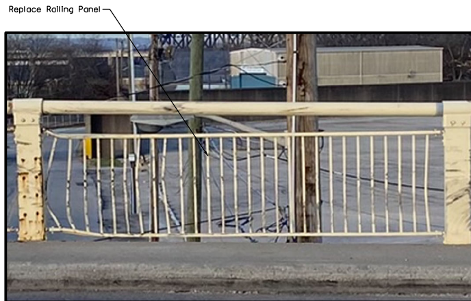
BRIDGE HANDRAIL REPAIRS (Span 27, Downstream Side)
